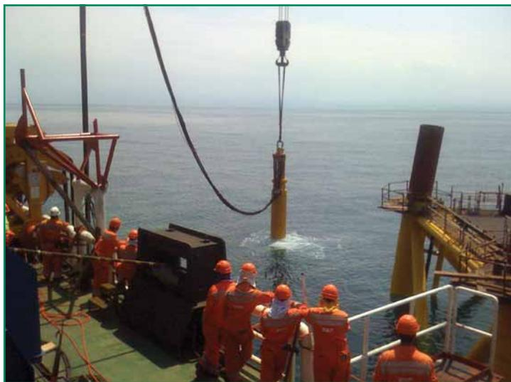
Underwater pile driving for an offshore oil platform.
