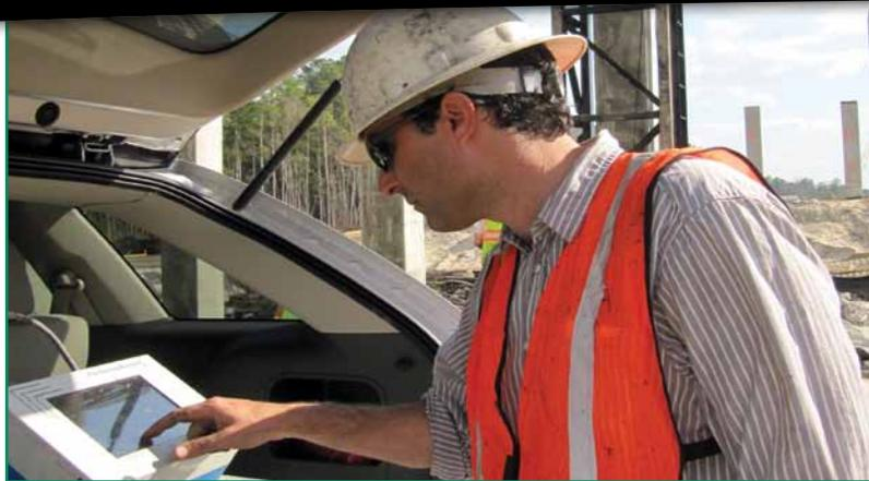
GRL Engineer monitoring the installation of driven concrete piles.
