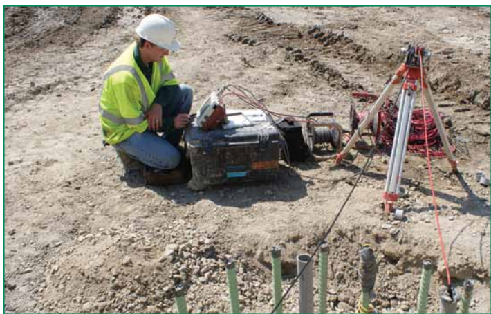
GRL engineer performing cross hole sonic logging.
