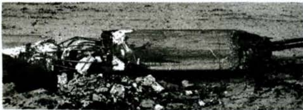
Fig. 3. Case 2, Damaged pile after extraction
