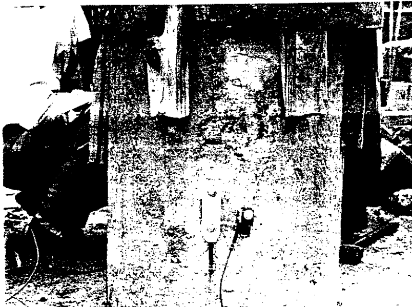
Figure 6: Strain transducer and accelerometer bolted to a pile
