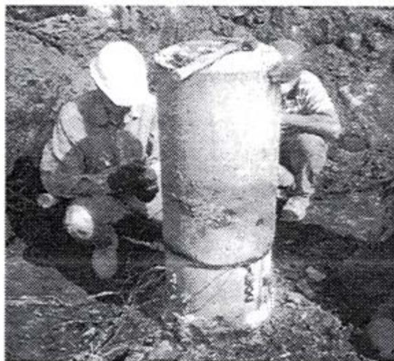
Fig 6: Attaching sensors to augercast pile
