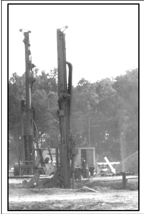
Fig. 2. Communication with adjacent holes was often evident during drilling.
