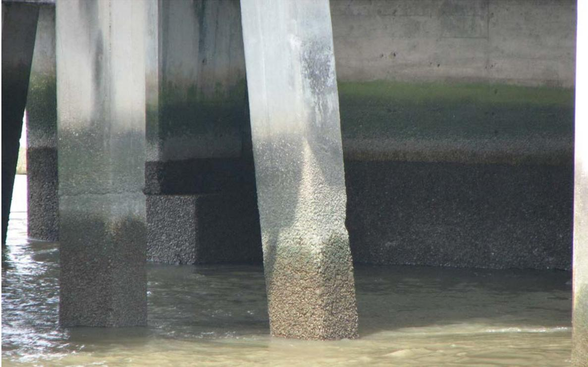
Figure 3-12 Concrete surface abrasion and deterioration in tidal zone (courtesy of Moser 2011).
