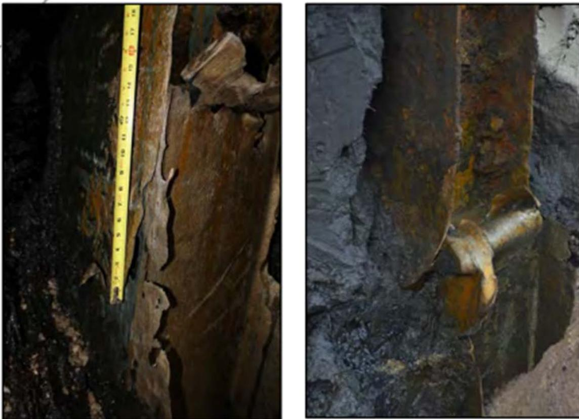
Figure 3-10 Corrosion and resulting buckling of foundation pile (courtesy Wisconsin Department of Transportation).
