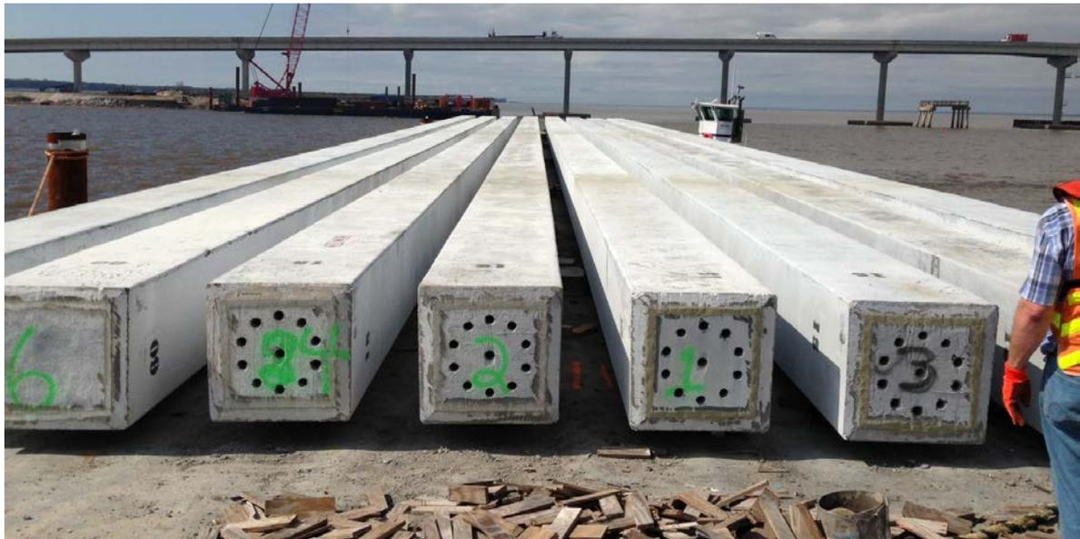
Figure 6-21 Square prestressed concrete piles.
