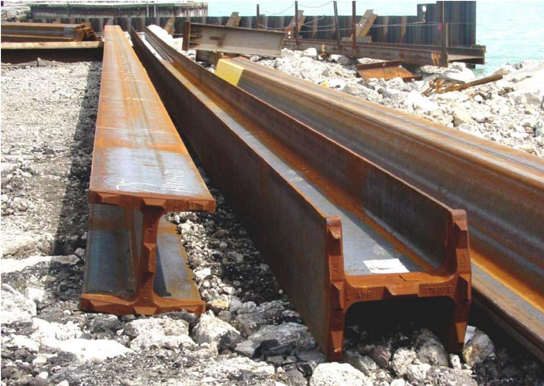
Figure 6-10 H-piles with driving shoes.
