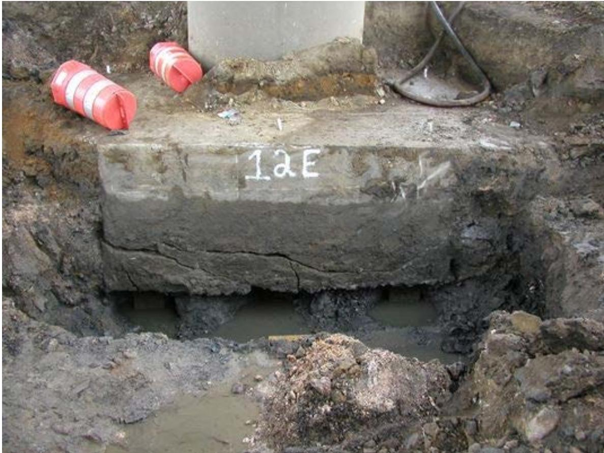
Figure 3-15 Cracked pile cap from lateral soil movements (courtesy DeIDOT).
