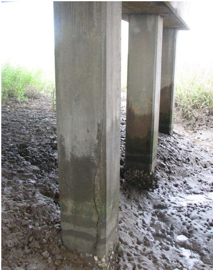
Figure 3-11 Concrete pile damage from corrosion effects on concrete pile reinforcement (courtesy of Moser 2011).
