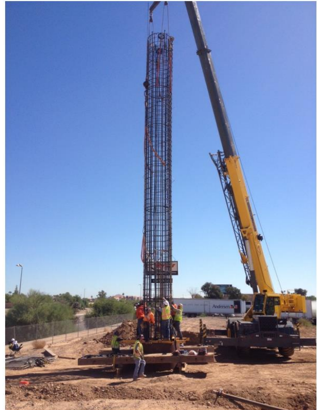
Figure 4. Photo of rebar cage for TS-2
