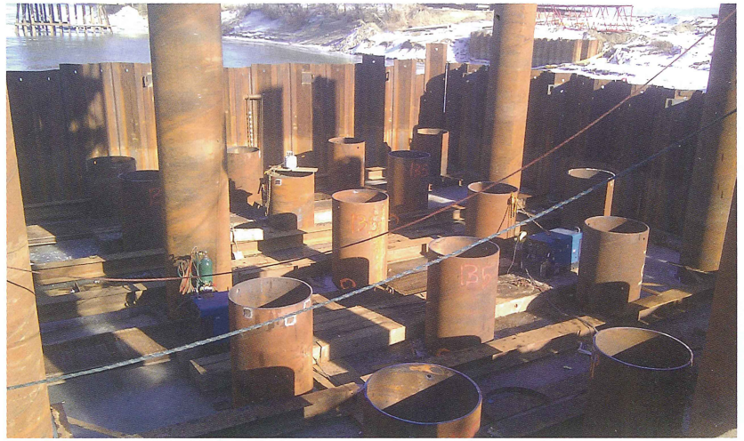
Each pier consisted of 30 open end pipe piles
