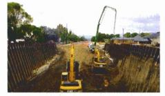
constructed on common abutments cast on spread footers supported by deep foundation piling. A Pile Driving Analyzer® and CAPWAP software (equipment and services provided by GRL Engineers, Inc.) was utilized to develop pile driving criteria and reduce excessive pile installation for all piles installed on the project.
