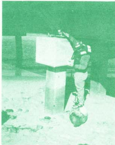
PIT Test on an existing bridge foundation; photograph by Mohamad Hussein, GRL Florida
