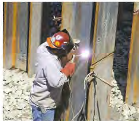
A construction worker welding the piles.
