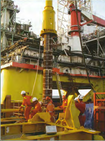
Dynamic pile testing offshore – PDA in the foreground
