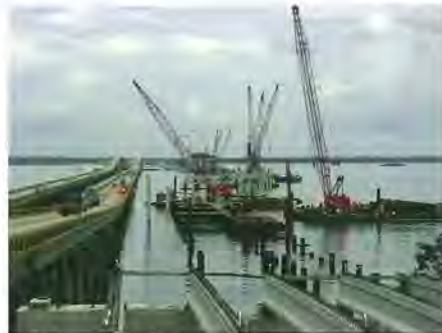
Bridge over Escambia Bay
