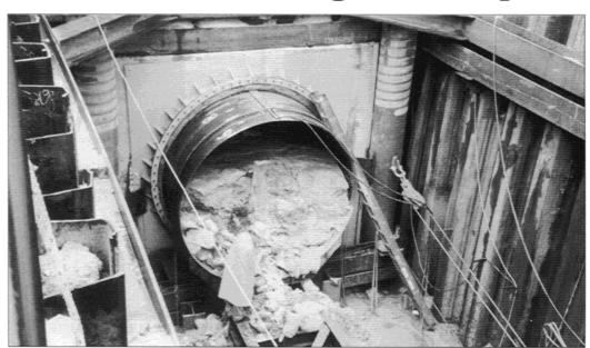
DYNAMIC TESTING techniques developed for pile driving have been used to monitor driving of a horizontal steel casing under a road and railway in Tampa, Florida.
