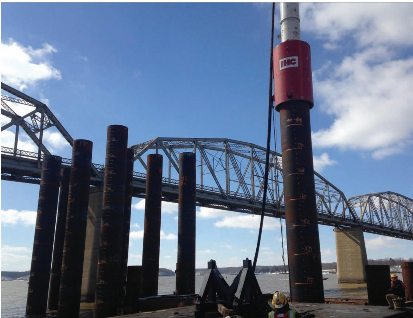
capacity evaluated during pile installation, however, may not fully represent the pile response in the static service condition. The high inertia of the soil prevents plugging during driving. The pile 'cookie cuts' its way into the ground, making installation to design penetration relatively easy but reducing end bearing during driving.
