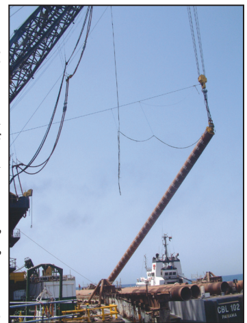
Pile being lifted - offshore oil platform in the Persian Gulf
