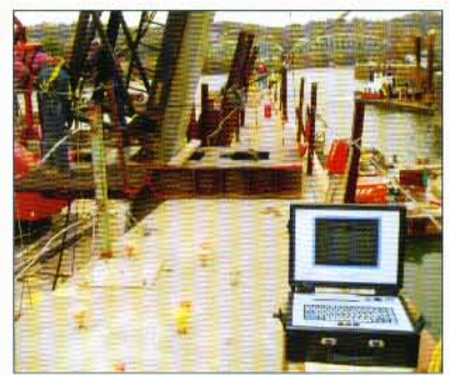
PDA on Charleroi Locks and Dam project
