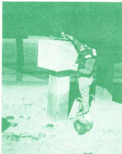
PIT Test on an existing bridge foundation; photograph by Mohamad Hussein, GRL Florida
