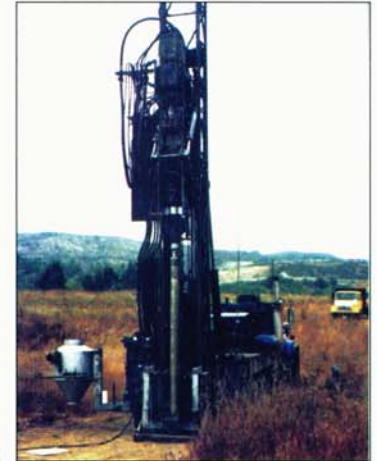
PDA monitoring of the Becker test improves its accuracy.
