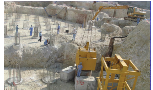
Foundations for Convention Tower, Qatar
