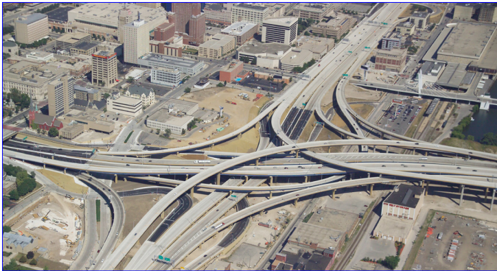
Marquette Interchange, completed project. Photo by WisDOT Marquette Interchange Project Team
