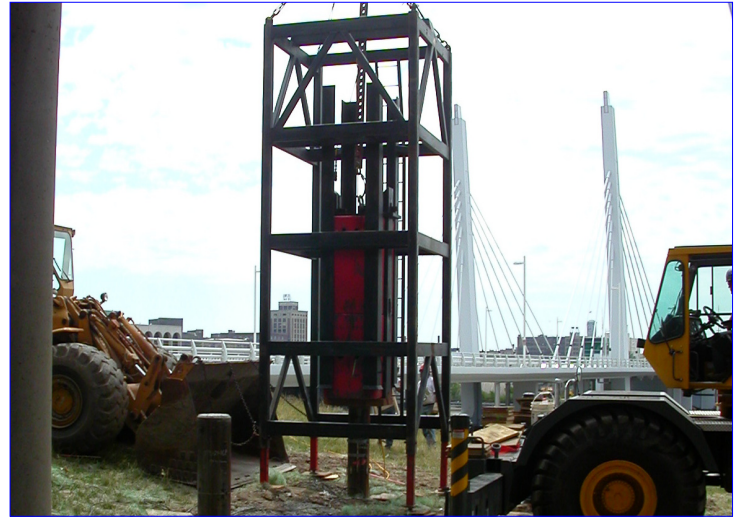
GRL's APPLE system was used on re-strike Dynamic Load Tests.
