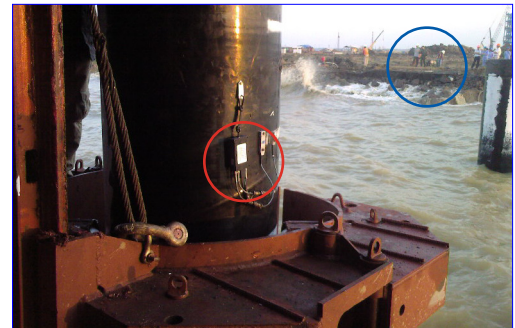
Red circle: Wireless sensors attached to pile; Blue circle: Engineers conducting the test with the PDA model PAX
