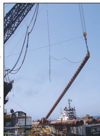
Pile being lifted - offshore oil platform in the Persian Gulf
