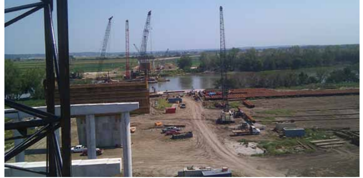
Aerial view of US 34 Bridge over the Missouri River.
