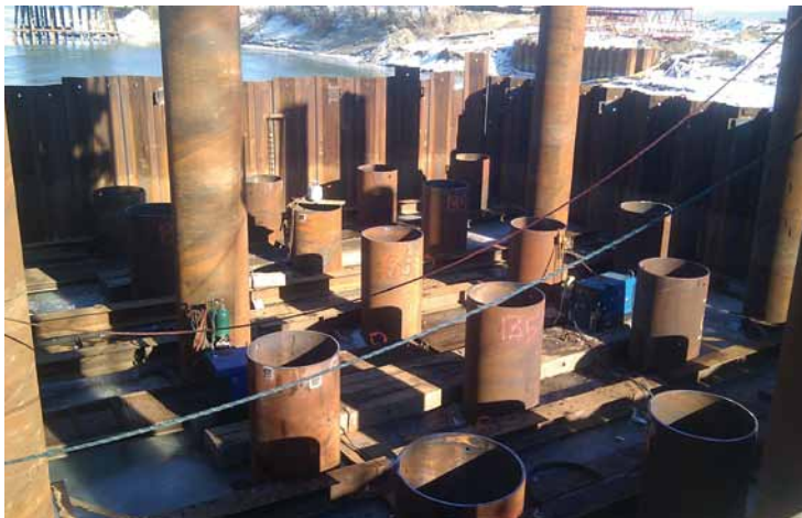
Each pier consisted of 30 open end pipe piles.
