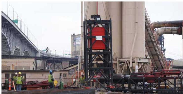
APPLE testing on large H piles, Innerbelt Bridge Project, Cleveland, OH
