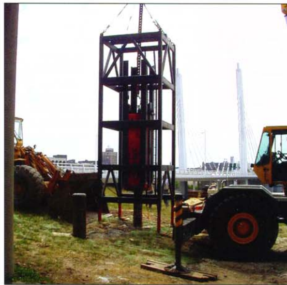
APPLE Testing near the 6th St. Viaduct
