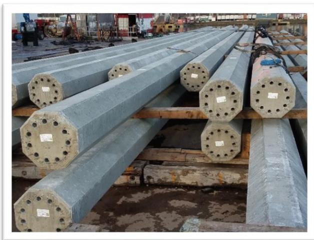
Individual piles range in length from 69.5 to 170.5 feet, and the required ultimate capacities range from 1,016 to 1,720 kips. It is estimated that 1,519 jobs in Washington State are somehow connected to the movement of cargo through this container terminal. The upgrades to Pier 4 will increase the cargo throughput, providing an opportunity to increase the number of jobs associated with the terminal over time.
