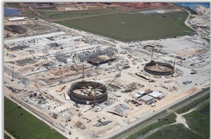
Corpus Christi Liquefaction Project April 2016
