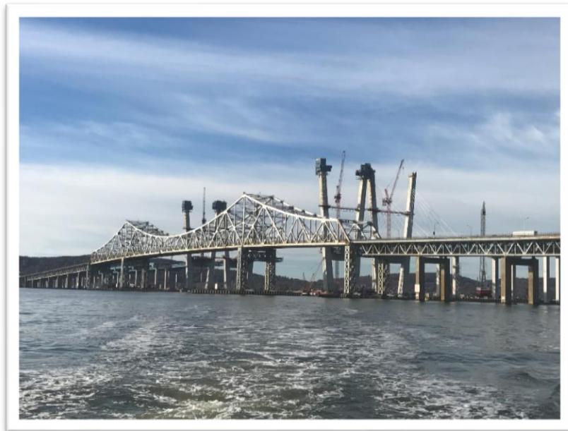
Construction of the new Tappan Zee Bridge in the background
