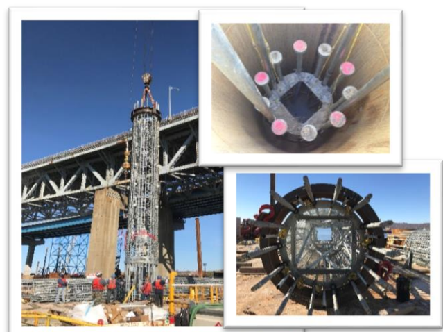
Construction of a 96-inch diameter drilled shaft
