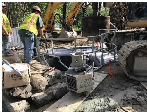
*SQUID ready for sediment thickness inspection*
