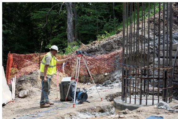
*Crosshole Sonic Logging performed on shafts*
