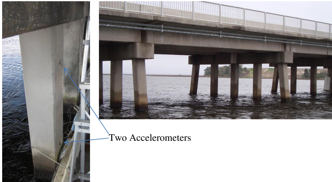
Figure 6. Photos of the Bridge, Bents, Pile and Locations of Accelerometers
