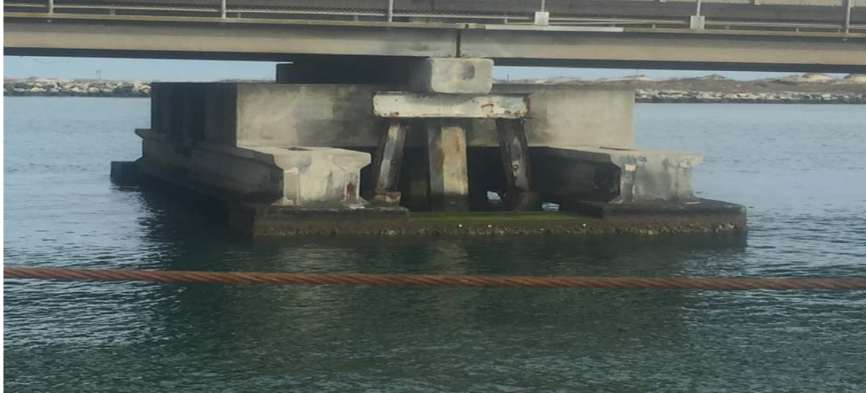
Figure 1. Typical underpinning of original bridge bent.
