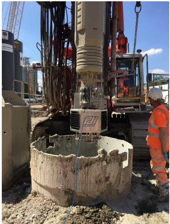
**Figure 3.** Shaft Quantitative Inspection Devices (SQUID), Ref. [4]
