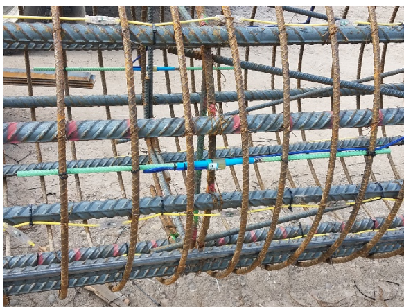
TIP Wires and Strainmeters on Reinforcing Cage
