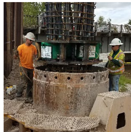
Bi-Directional Static Load Test Jack Assembly in Reinforcing Cage
