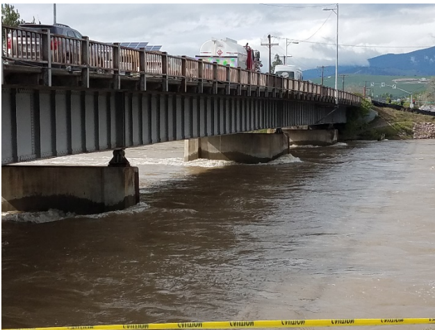
Existing 2-lane bridge
