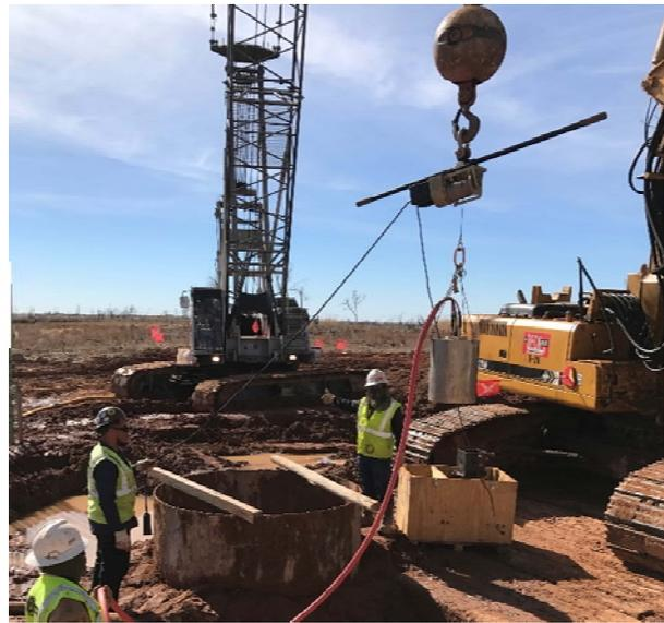
b) Mini-SID lowered into the drilled hole
