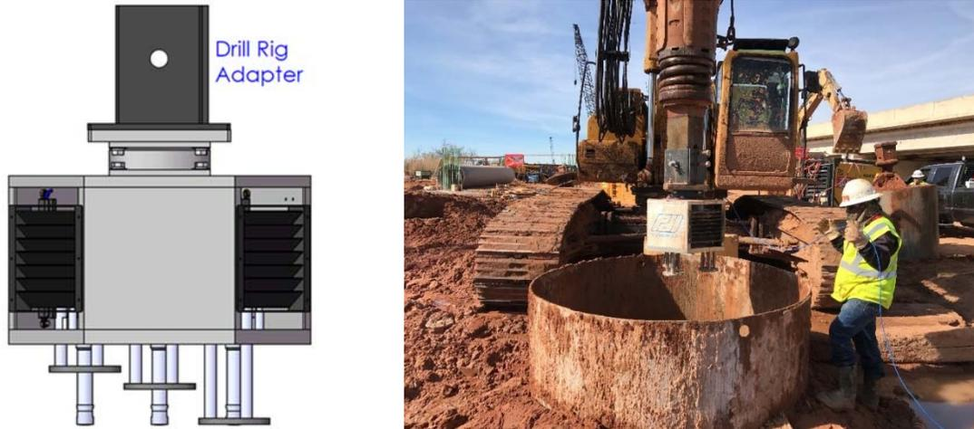
**Figure 3.** Shaft Quantitative Inspection Device
