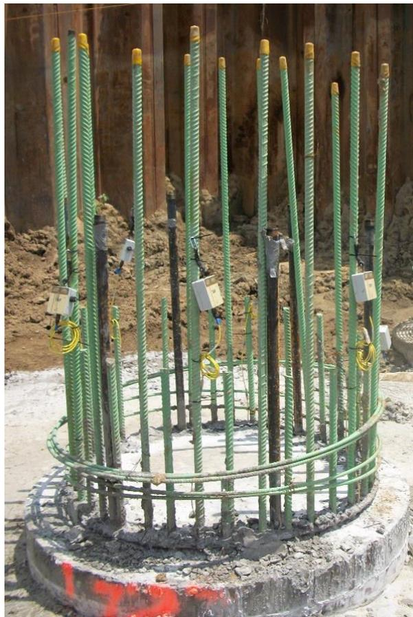
**Figure 1. Thermal wire cables attached to data loggers**
