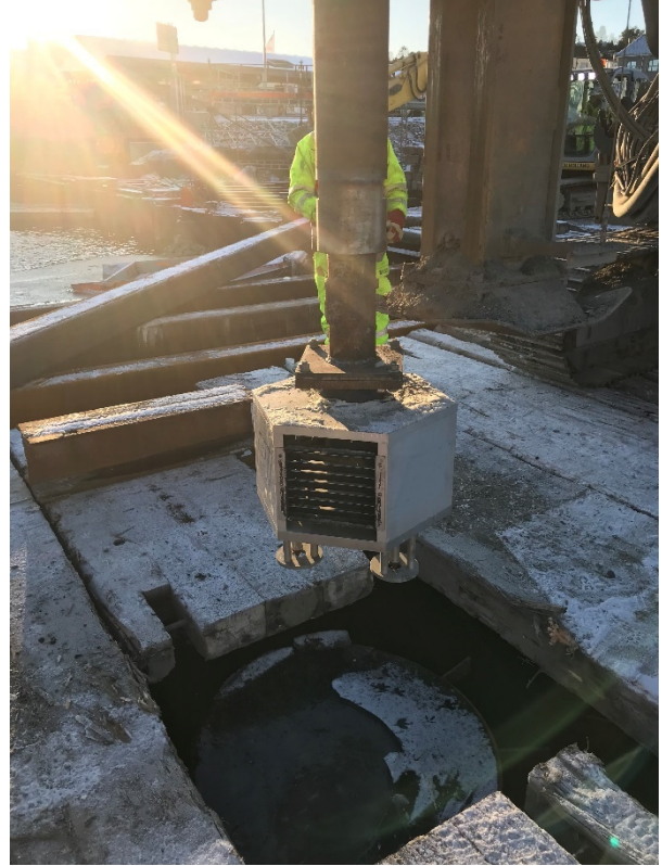
Figure 4. Testing procedure for Bent 2, Drilled Pile P02-05
