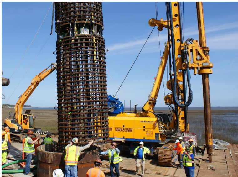
Lowering rebar cage into shaft for Bi-Directional Static Load Testing
