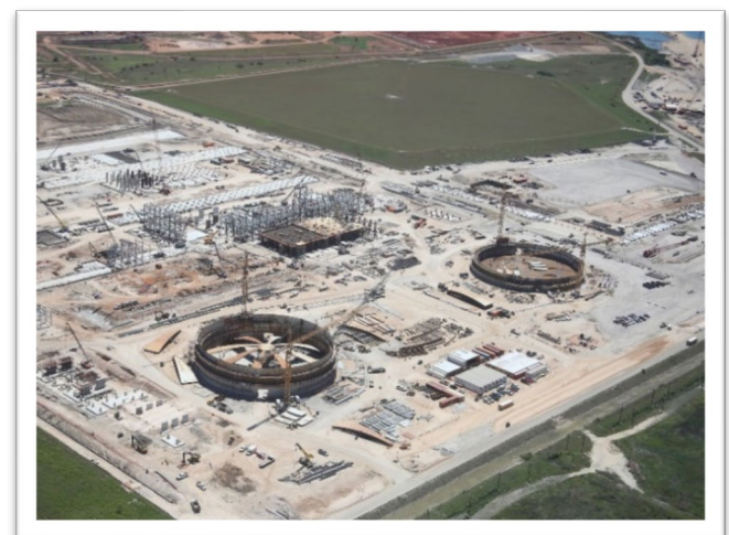
Corpus Christi Liquefaction Project April 2016
