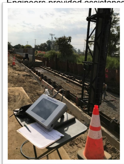
Dynamic Pile Testing
