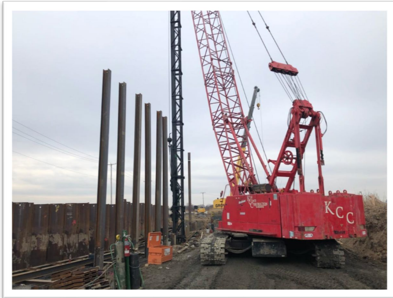
Driven Piles for the Hurricane and Storm Damage Reduction Floodwall Foundation
