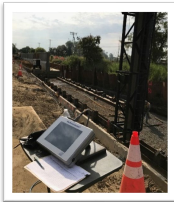
Dynamic Pile Testing (PDA)
