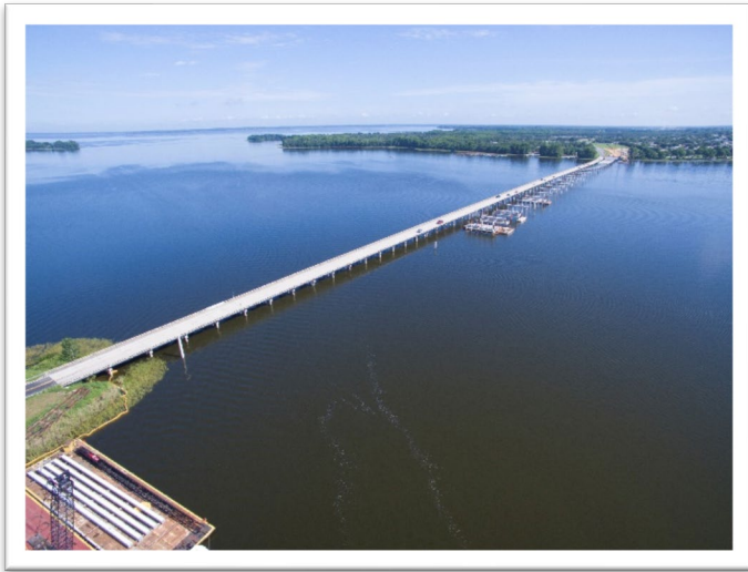
SR-19 during construction
