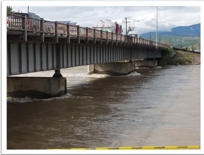
Existing 2-lane bridge
