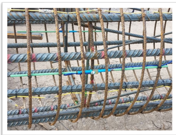
TIP Wires and Strainmeters on Reinforcing Cage
