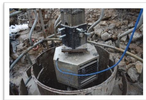
Drilled shaft base cleanliness evaluation being performed
