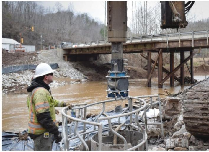
Shaft Profile and Verticality using the SHAPE
