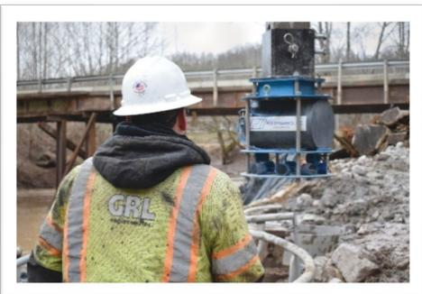
Drilled shaft profile / verticality evaluation being performed
