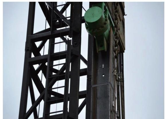
Figure 2. The ICE 66-80 hammer on the instrumented HP 46x304 pile.
