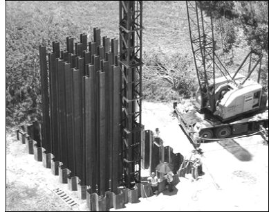
Figure 2: Pile driving at a bridge pier.
