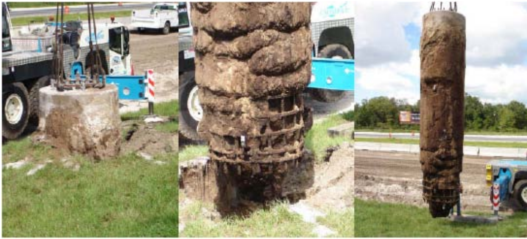
Figure 1-3a Exhumed shaft with compromised durability as well as structural and geotechnical capacity.
