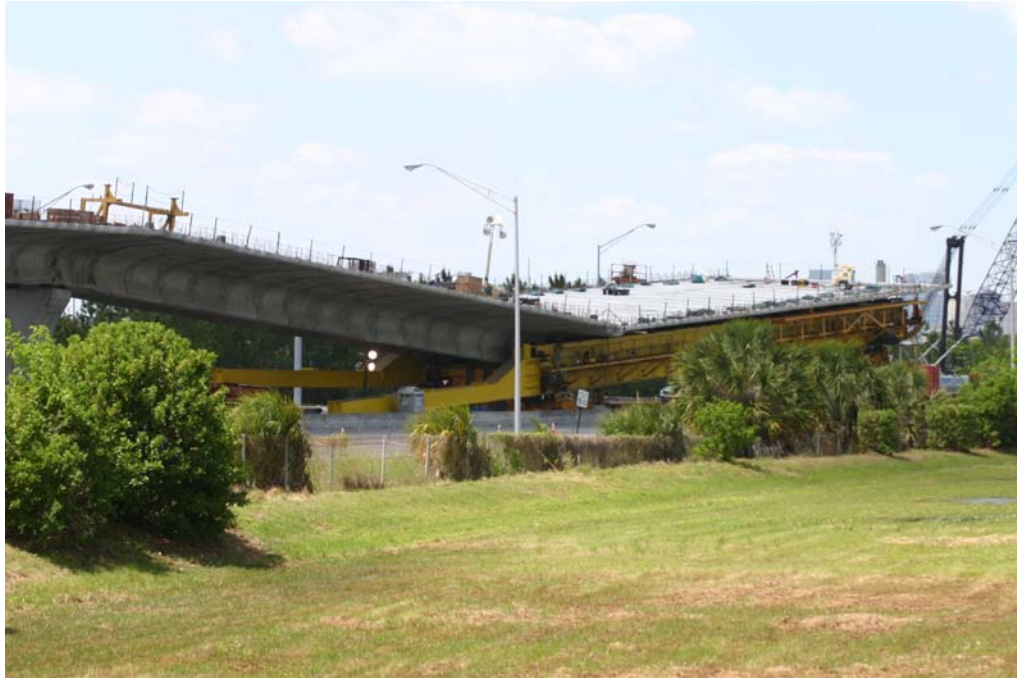
Figure 1-2 Bridge pier plunging failure from insufficient geotechnical capacity.
