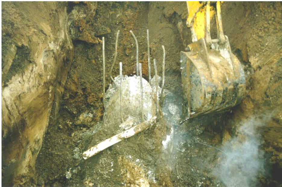
Figure 1-1 Drilled shaft failed during load testing at 1100 psi concrete stress.
