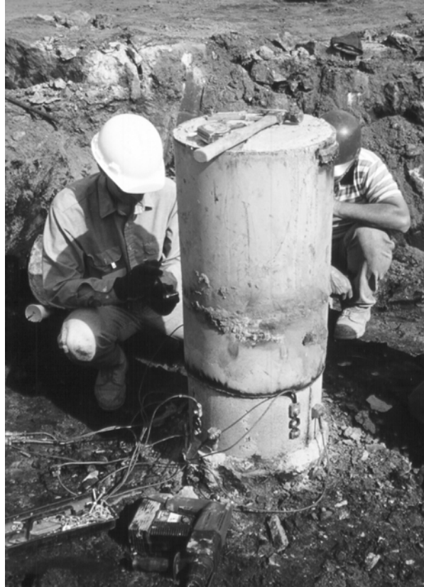
Figure 1: Test preparations with four strain transducers for a small drilled shaft.
