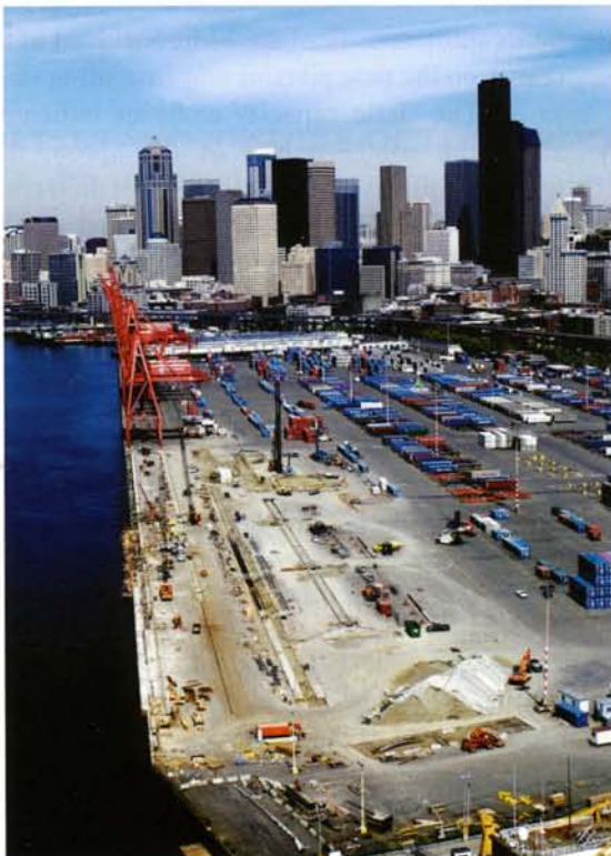
Figure 1 – Photograph of site
