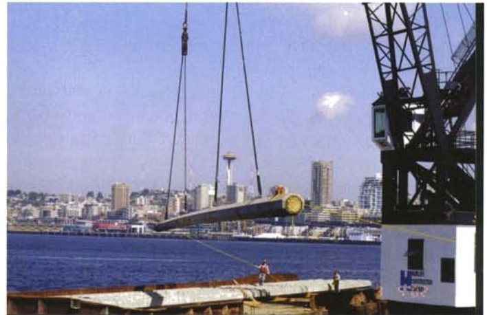
Figure 4 - Handling of 55-m-long concrete pile
