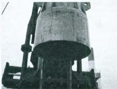
Fig. 1. Follower to steel pile connection
