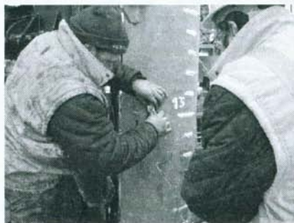
Fig. 3. Instrumenting the steel follower
