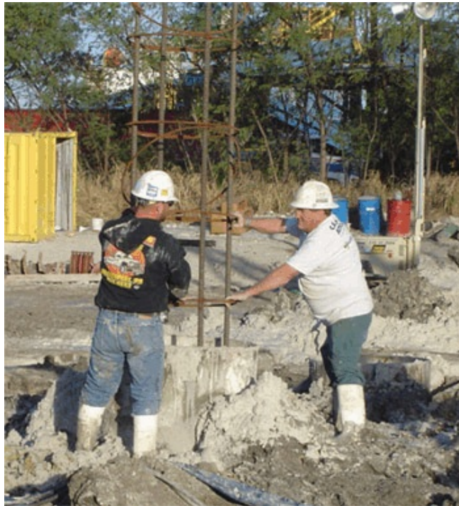
Figure 7-3. Cage Installation at the Port of Tampa
