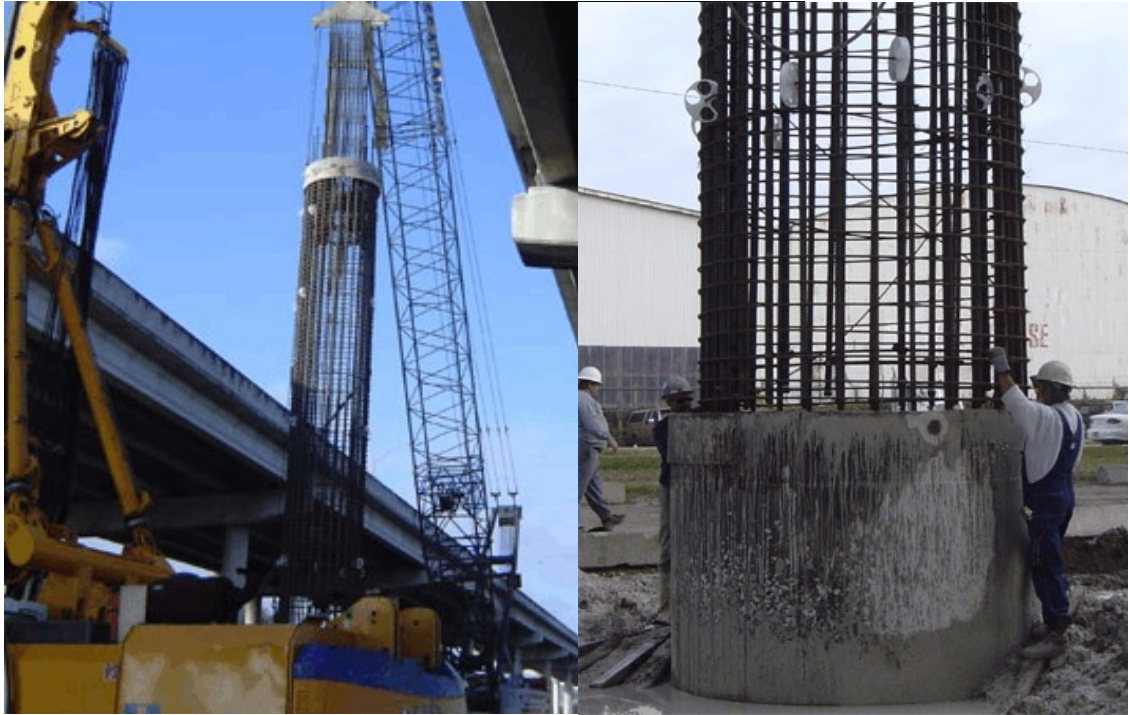
Figure 7-7. Mono-pier Cage Placement at the Crosstown Expressway
