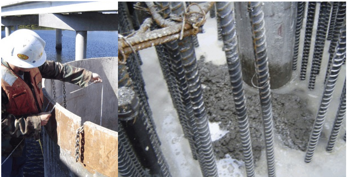
Figure 7-8. Head Differential Measurements at the Crosstown Expressway
