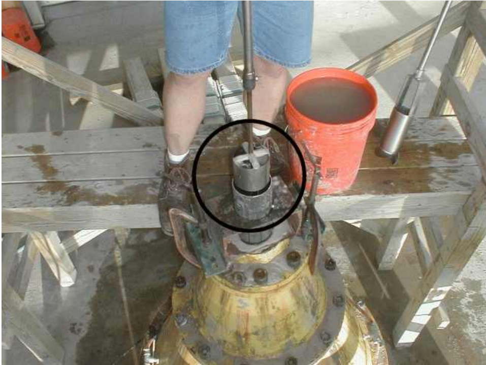
Figure 4-5. Clean-out Bucket Used to Finish Excavation
