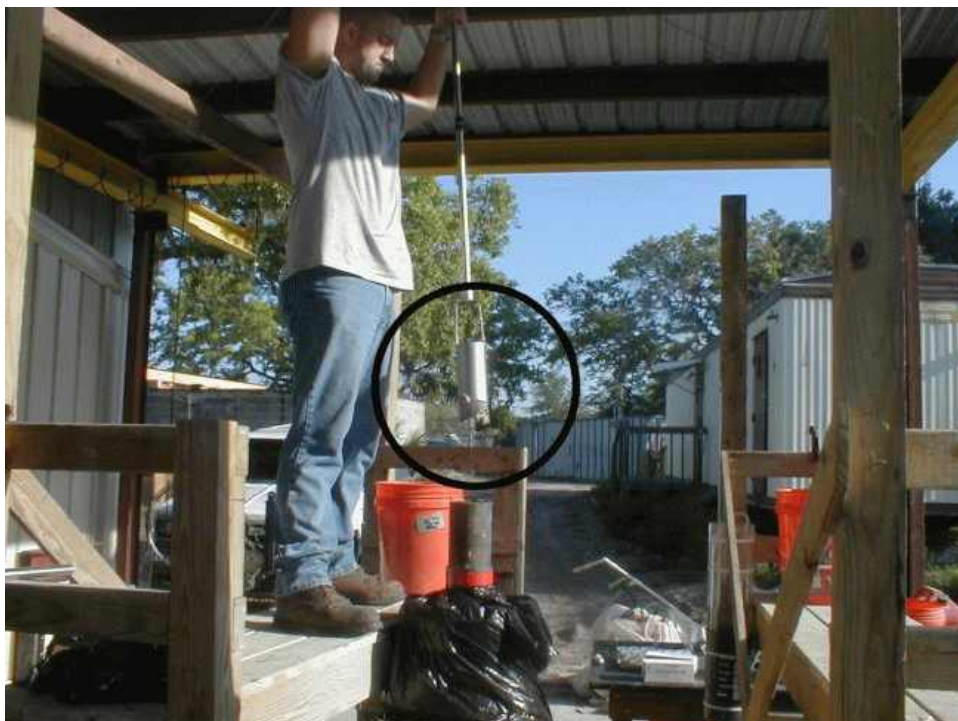
Figure 4-4. Primary Auger Tool Used to Excavate Most of the Shaft
