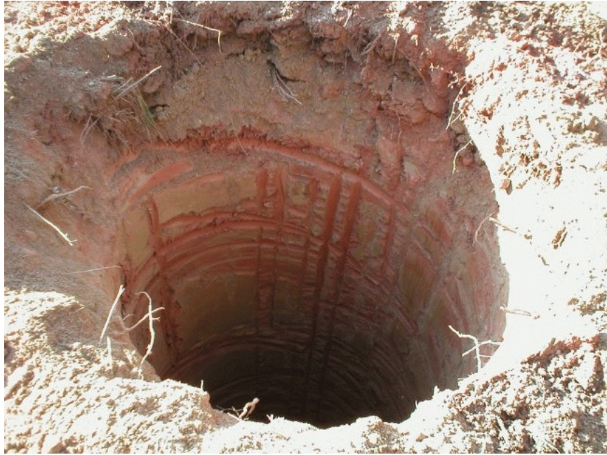
Figure 6-17. Dry Hole Drilling Was Used Because of Soil Conditions on Site
