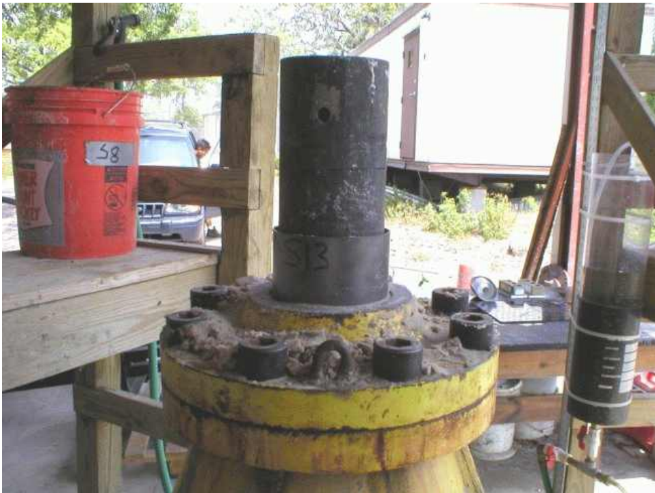
Figure 4-6. Permanent Casing Installed Around Temporary Casing
