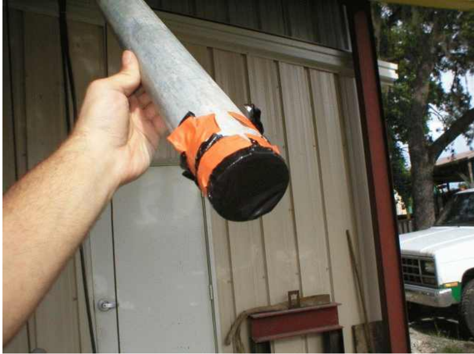
Figure 4-7. Tremie Plugged to Prevent Segregation
