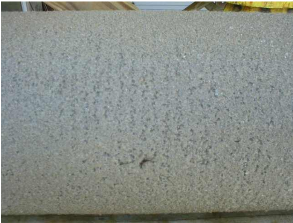
Figure 4-26. Porous surface noted during rapid casing extraction on Shaft S41
