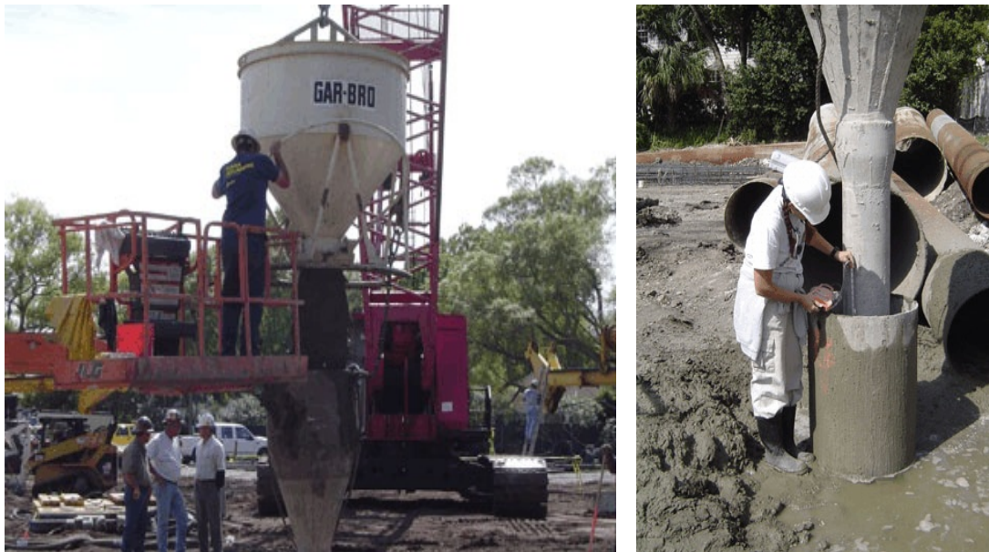
Figure 7-10. Alagon Bucket Pours (left) and Field Measurements (right)
