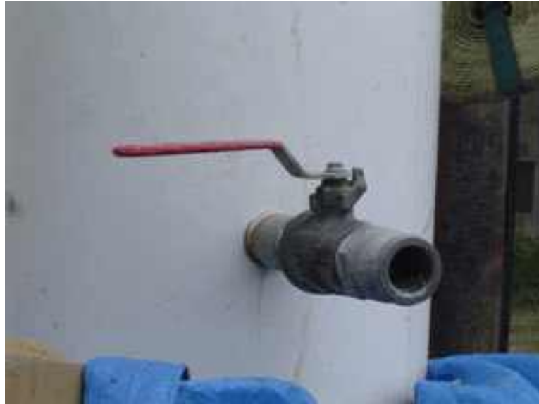
Figure 5-3. Intake Fitting
