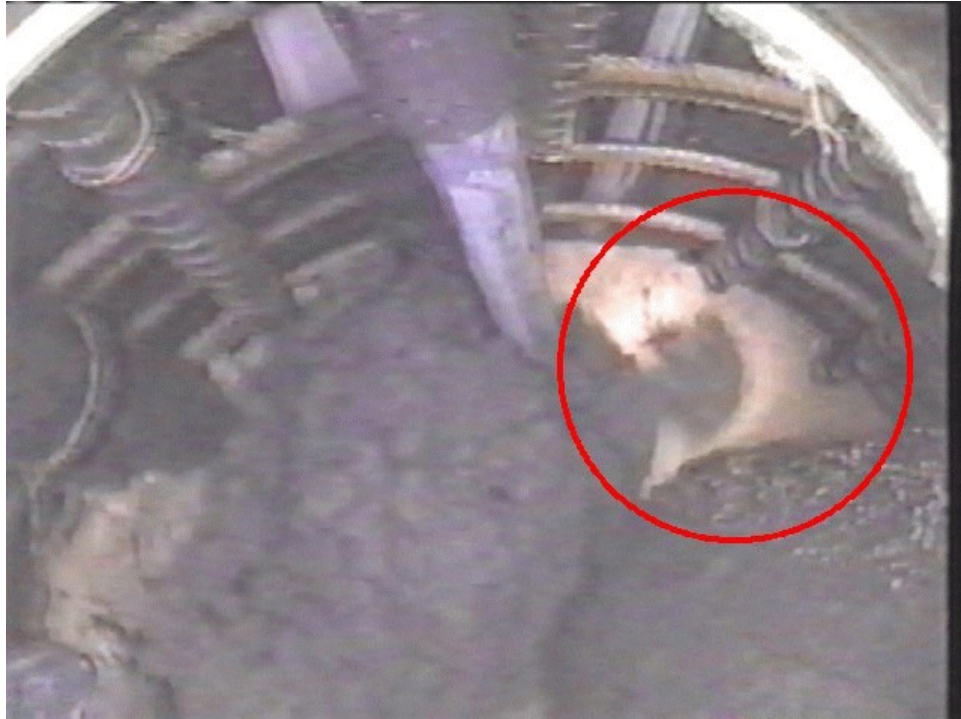
Figure 6-31. TS-3: Obvious Segregation and Bleed off of Mix Water During Pour
