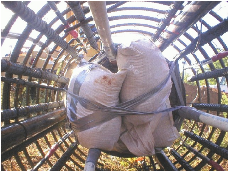
Figure 6-6. View of Toe Sand Bags from Inside the Cage
