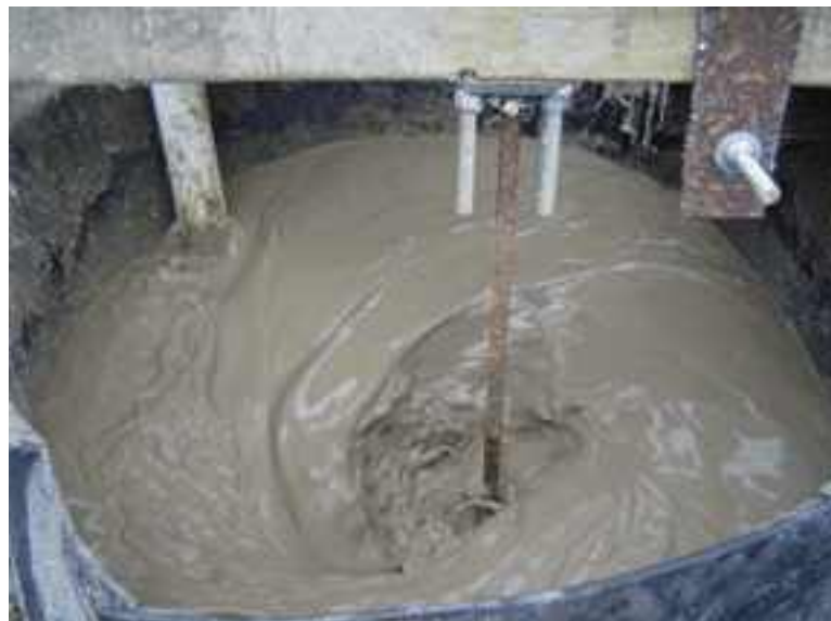
Figure 5-10. Mixing Slurry with Device
