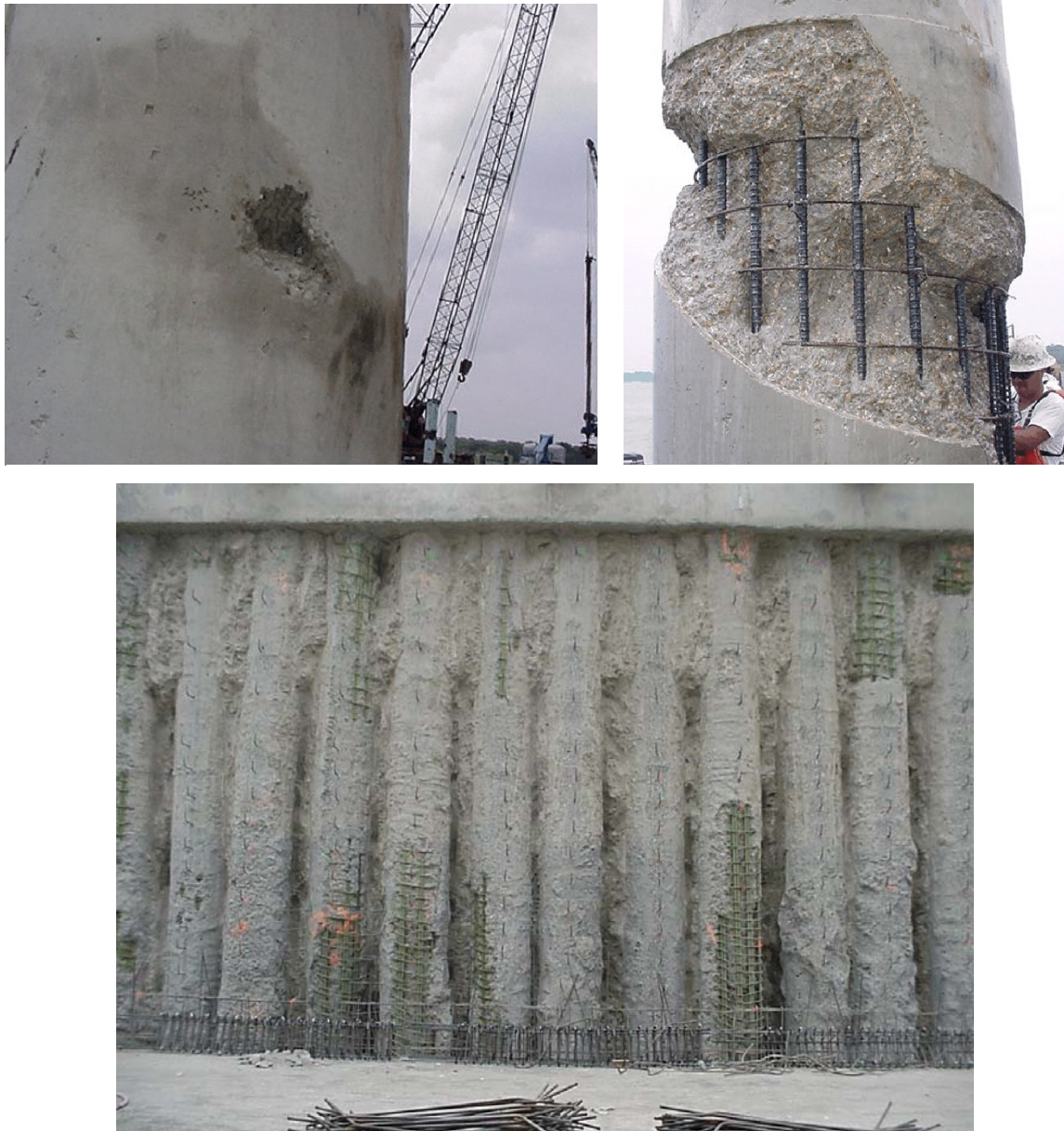
Figure 1-2. Anomalies in cased construction caused by concrete quality (top) and in slurry supported construction caused by bottom of excavation soil accumulation (bottom).
