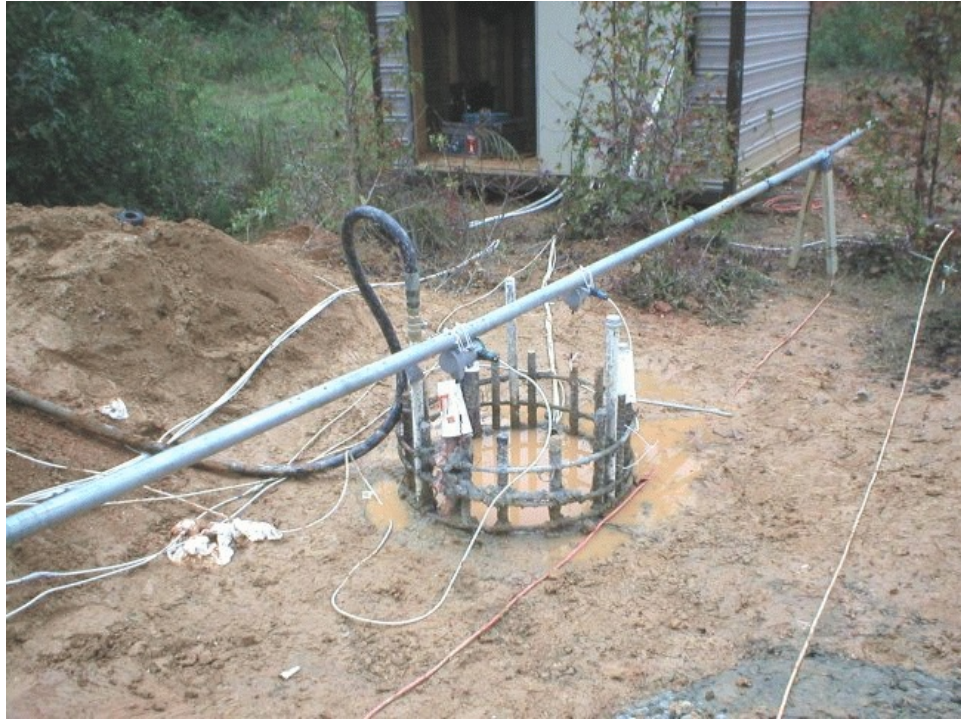
Figure 6-53. Post Grouting Operation Injects Grout to Shaft Tip
