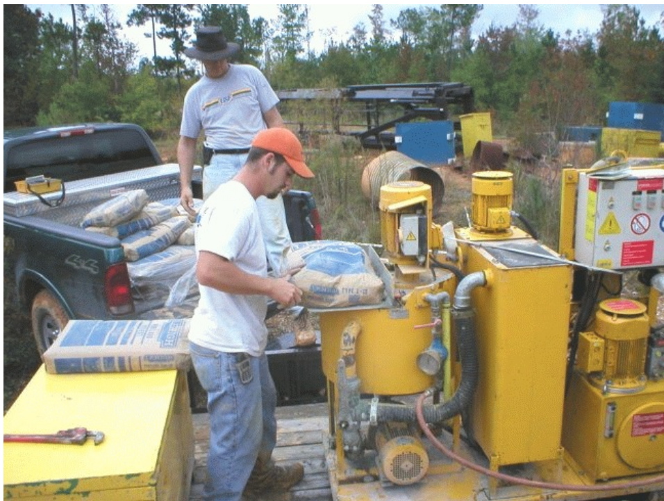
Figure 6-52. Mixing Grout in the Pump Prior to Post Grouting Each Shaft
