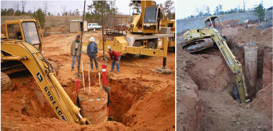
Figure 6-65. Soil Excavation for Shaft Removal
